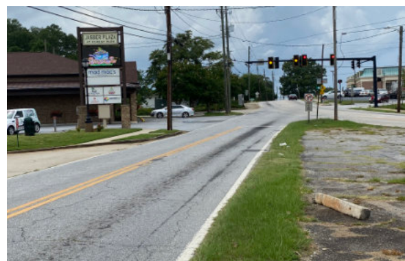
Lack of Sidewalk and Crosswalk on Courtney Drive
