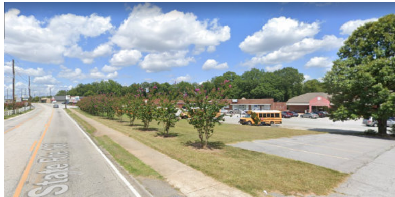
EXISTING MAIN STREET LOOKING WEST NEAR FOREST PRIMITIVE BAPTIST CHURCH
