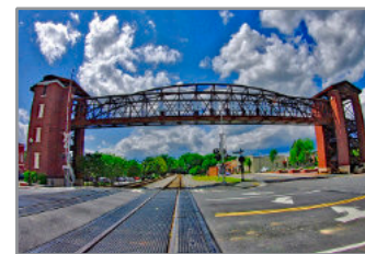
Pedestrian bridge on Forest Parkway
